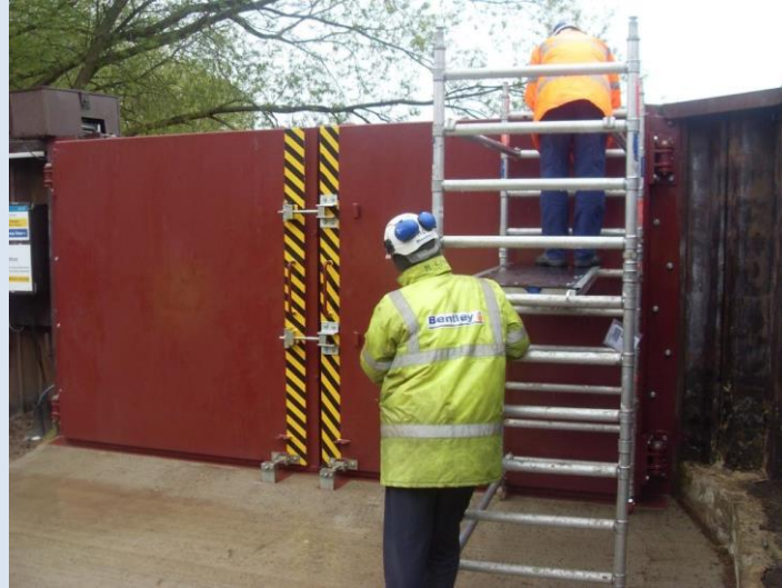
Croft on Tees 'off seat pressure' Double Leaf Flood Defence Gate
